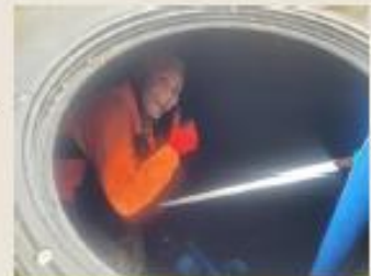
Ranger Christina Paterson cleaning out a Great Walk water tank. Photo by Nick Stinson DOC
