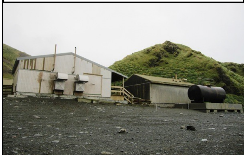
The two power houses
