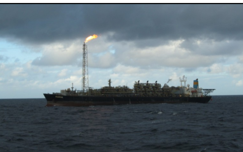
The FPSO (Floating Production Storage and Offtake) Raroa.
