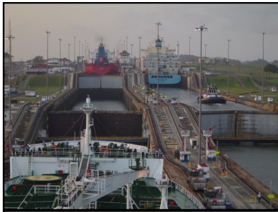
The three-stage Gatun Locks lifting ships up to Lake Gatun.
