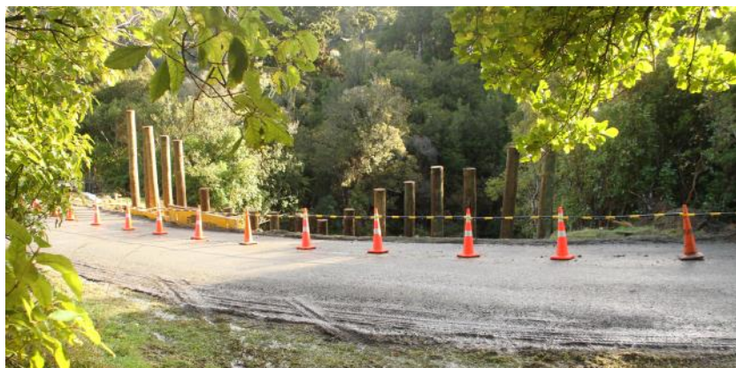
Roadwork at the Horseshoe Bay slip. Photo from Greg Northe
